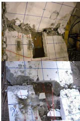
Fig. 9: Crushing of concrete in compression face.
